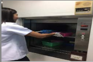
Send to elevator
